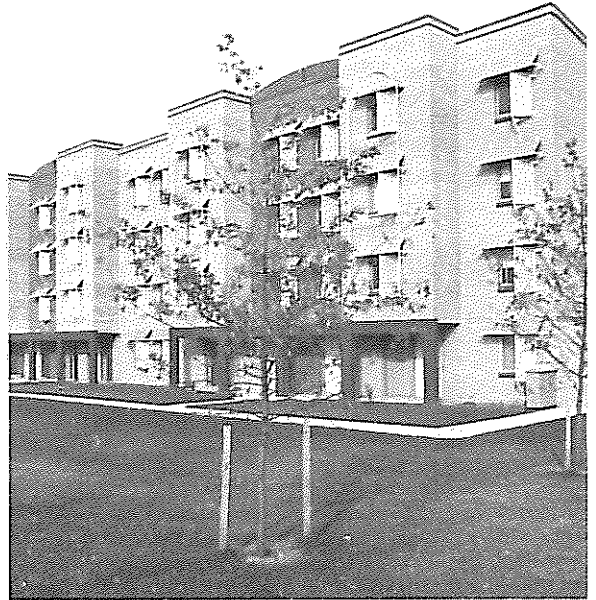
AIS Halls of Residence
